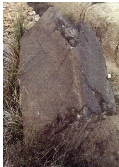
Fig. (6): Parts of basalt show cracking & severe weathering. Dense plant vegetation indicates new surface water at Tell Basta.
