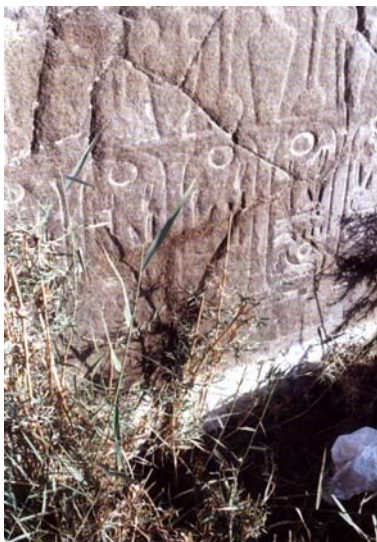
Fig. (5): Basaltic block showing white salt efflorescence at its base & coarse single cracks, Memphis.
